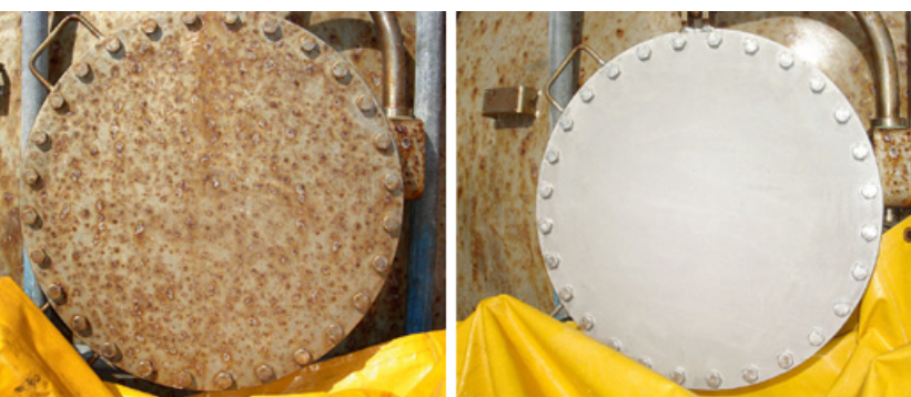
Before and after cleaning.
